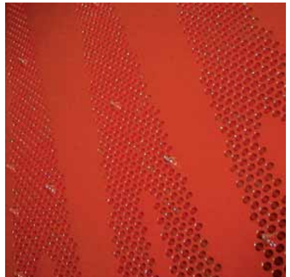
Tube inlets coated with Plastocor® Inlet
