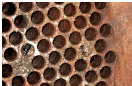
An unprotected tube sheet exposed to galvanic corrosion
